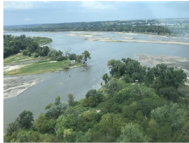
Platte River breach flows over Plattsmouth's water treatment plant - USACE
