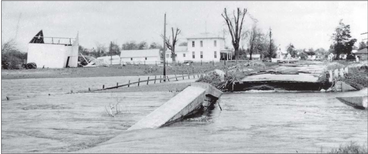
Photo 1-2. Heavy rains produced this flooding that destroyed a rural bridge, and a tornado did major damages to the nearby farm and its trees.
