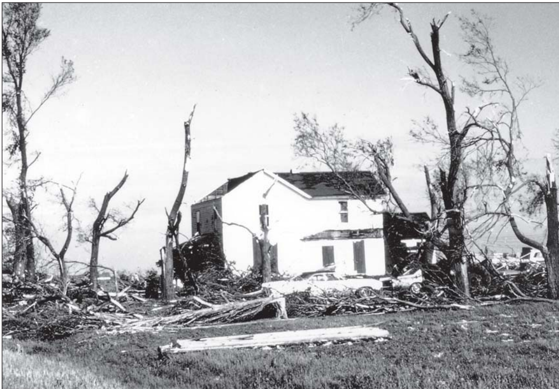
Photo 4-2. A farm house and trees destroyed by a tornado.
