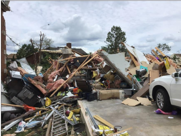
Tornado Damage in Woodridge, IL: June 20, 2021 Courtesy: Chicago, NWS
