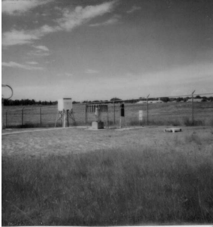
Figure 8. Cheyenne, Wyoming, National Weather Service instruments located at the municipal airport in August 1987. The Cotton Region shelter and the rain gages can be seen in this photograph taken 20 feet from the office building looking north. From the station history files at the National Climatic Data Center.
