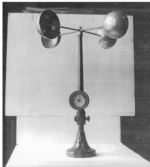
Figure 19. Four-cup Anemometer, Seattle 1925 Source: Seattle Museum of History and Industry
