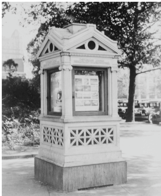
Figure 34. Kiosk, Unknown Location Source: NOAA Photo Library
