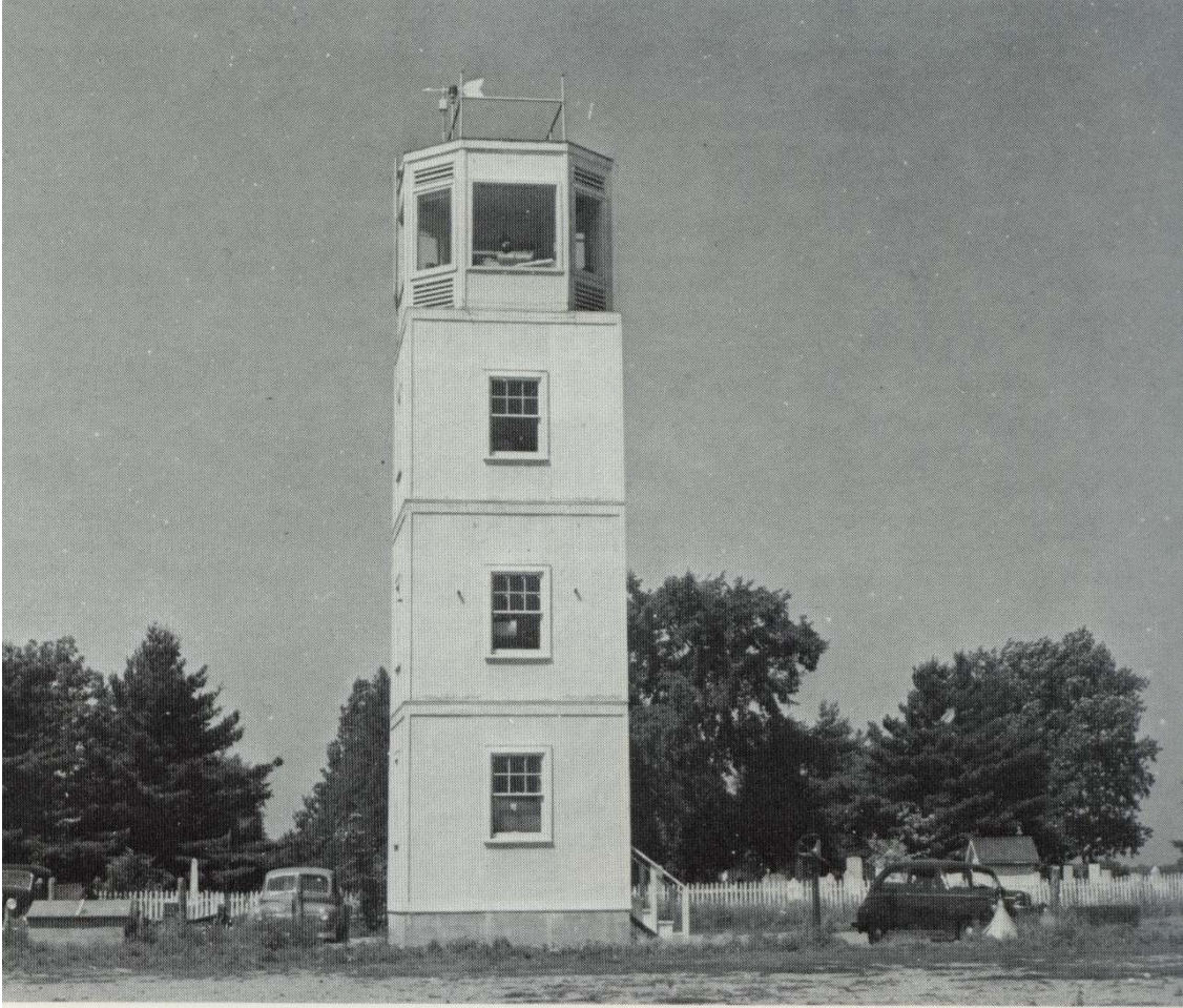
Figure 9. The Air Traffic Control Tower at the Burlington, Vermont Municipal Airport circa mid-1940's. The Tower was 42 feet tall containing 105 steps. Photograph courtesy the Board of Airport Commissioners, Burlington International Airport.
