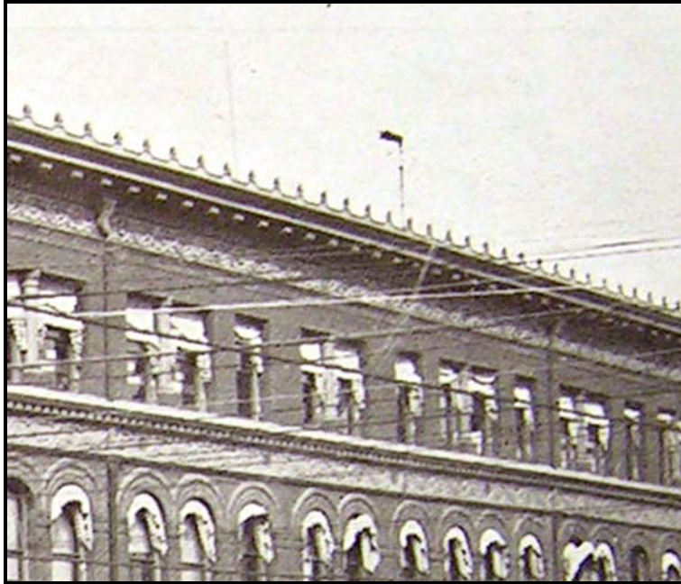
Figure 30. Enlargement of Figure 29 showing the wind vane on top of the Hicks Building. View is northwest. Courtesy of the San Antonio Conservation Society Foundation.
