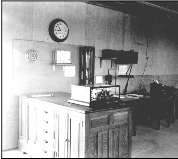
Figure 41. Photograph of the Weather Bureau office in the east lean-to, Hangar No. 2, Municipal Airport (22 August 1942) showing the mercurial barometers and barograph. View is northwest. From the official station history files at the National Climatic Data Center.
