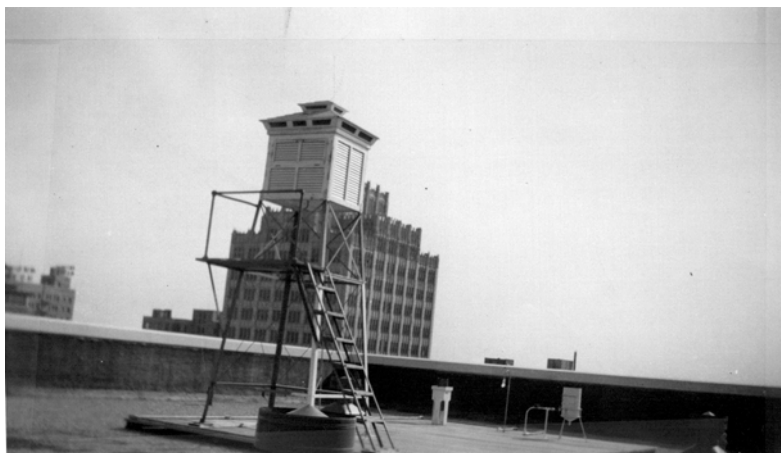
Figure 12. A view of the weather instruments above the U.S. Court House, Austin, Texas, in November 1936. The view is looking southeast.
