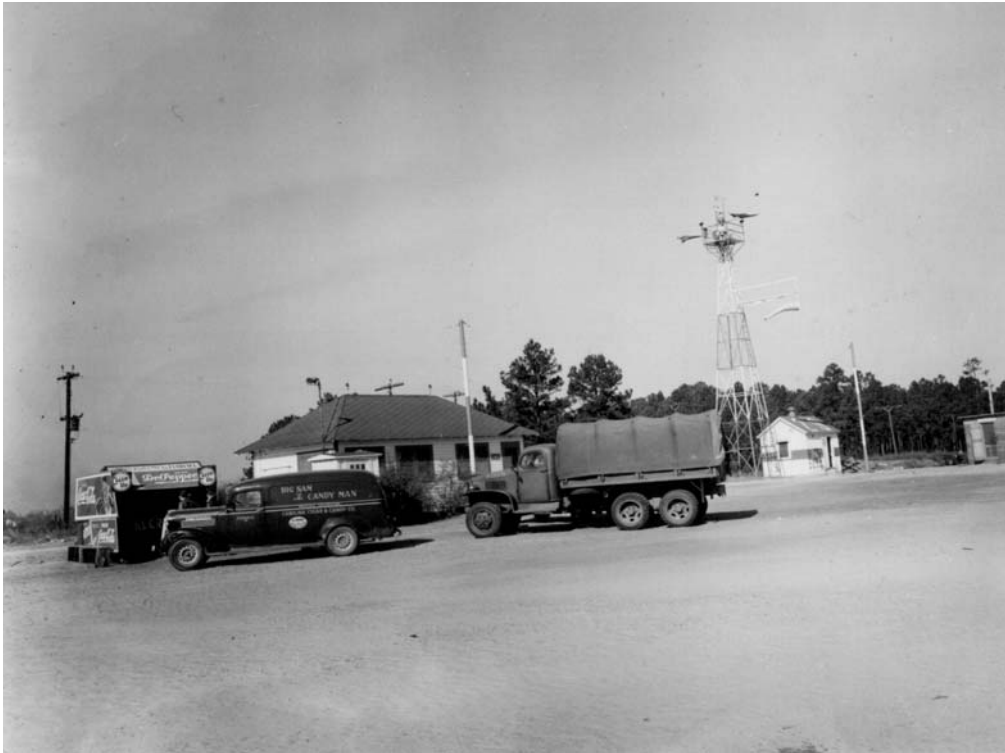
Figure 4. Northwest view of Civil Aviation Administration Building, Florence, South Carolina, airport, 25 November 1941. Wind instruments were mounted on tower.
