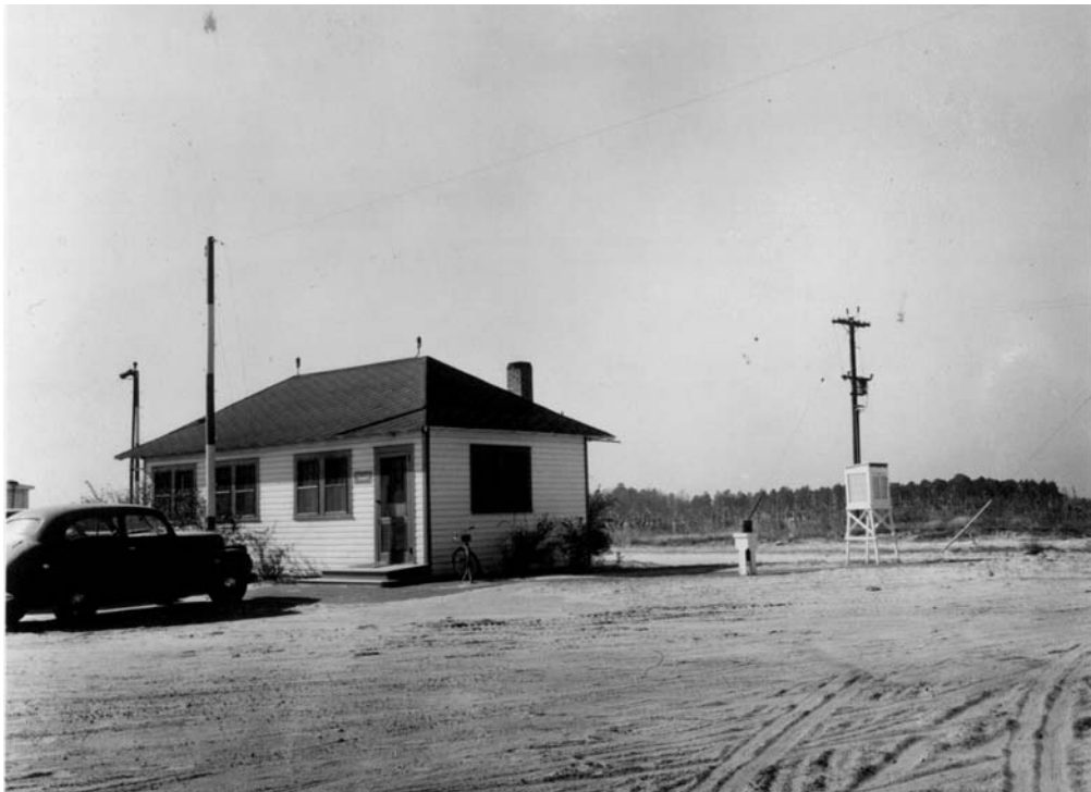
Figure 3. Southwest view of Civil Aviation Administration Building, Florence, South Carolina, airport, 25 November 1941.
