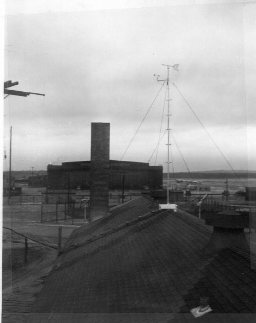
Figure 29. The wind equipment at Building 317, Columbia Municipal Airport, Columbia, South Carolina, 20 February 1947. Camera is facing east southeast. Source: Official station history files at the National Climatic Data Center.
