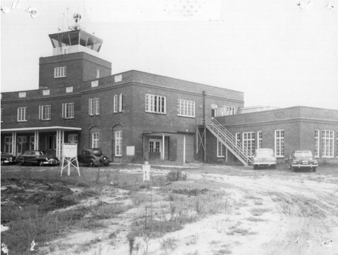
Figure 12. The Charleston, South Carolina airport new Administration Building on 22 August 1949. The instrument shelter and the rain gage are shown in the foreground. Wind instruments were on the roof of the Tower. The Weather Bureau office was at the top of the stairs. Source: Official station history files, National Climatic Data Center.
