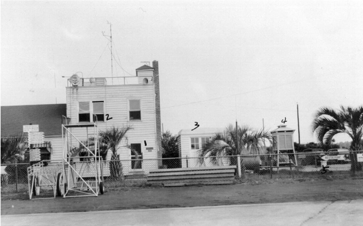
Figure 8. The Administration Building at the Charleston, South Carolina, airport on 24 May 1941. View looking southeast. Source: Official station history archives, National Climatic Data Center.
