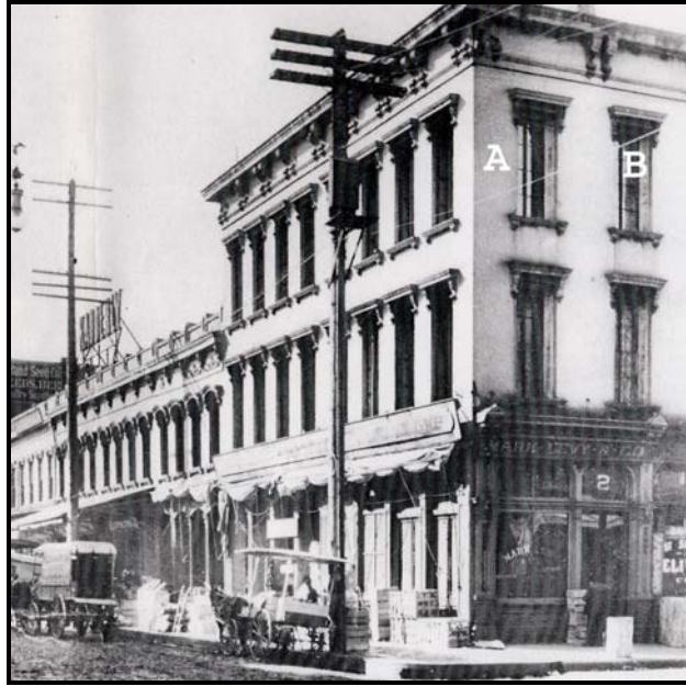
Figure 5. The Parrish Building (tallest building on right side of picture; circa 1899) at the southwest corner of Washington and Front Streets that housed the Signal Service office Dec 21, 1872 – Jan 1, 1878. View is southwest with Front Street located to the left of the building and Washington Street intersecting from the right. The Signal Service office was located on the top floor, in the northeast part of building (indicated by letter “A” in the photograph). The three windows were on the east wall of the Signal Service office with the two windows to the right of the building corner the northern wall of the office. The temperature shelter was mounted outside the second window to the right of the building corner (indicated by letter “B”). From the Oregon Historical Society.
