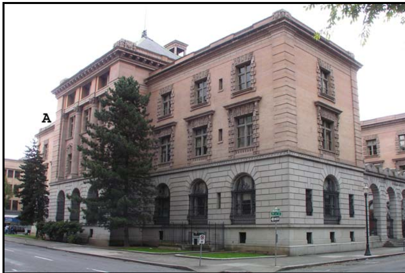
Figure 9. The U.S. Custom House Building (photo taken Sep 2004) at Davis-Everett on Park. View of the building looking southeast from the North Park. Instrument shelter and rain gages were located on flat part of roof near point “A.”
