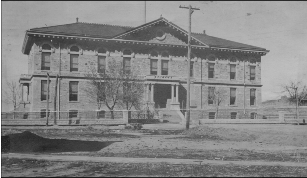
Figure 10. Federal Building located at Federal and Lincoln Avenues (circa 1908). View is looking north. Weather Bureau office was located on the 2nd floor (top floor). On Sep 24, 1908, the Weather Bureau office moved to the middle, or 1 st floor (building comprised of three floors-basement, first floor, and second floor, i.e., outside stairs empty onto the middle, or first floor). Weather instruments were located west northwest of the building (to the left and out of the photo; see Figure 11). From the official station history files at the National Climatic Data Center.
