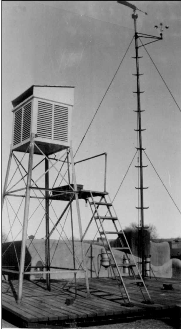
Figure 18. Close-up photograph of weather instruments on roof of the Post Office (circa 1932). View is looking northwest. Station records indicate the size of the instrument platform was 20 feet by 20 feet. From the official station history files at the National Climatic Data Center.
