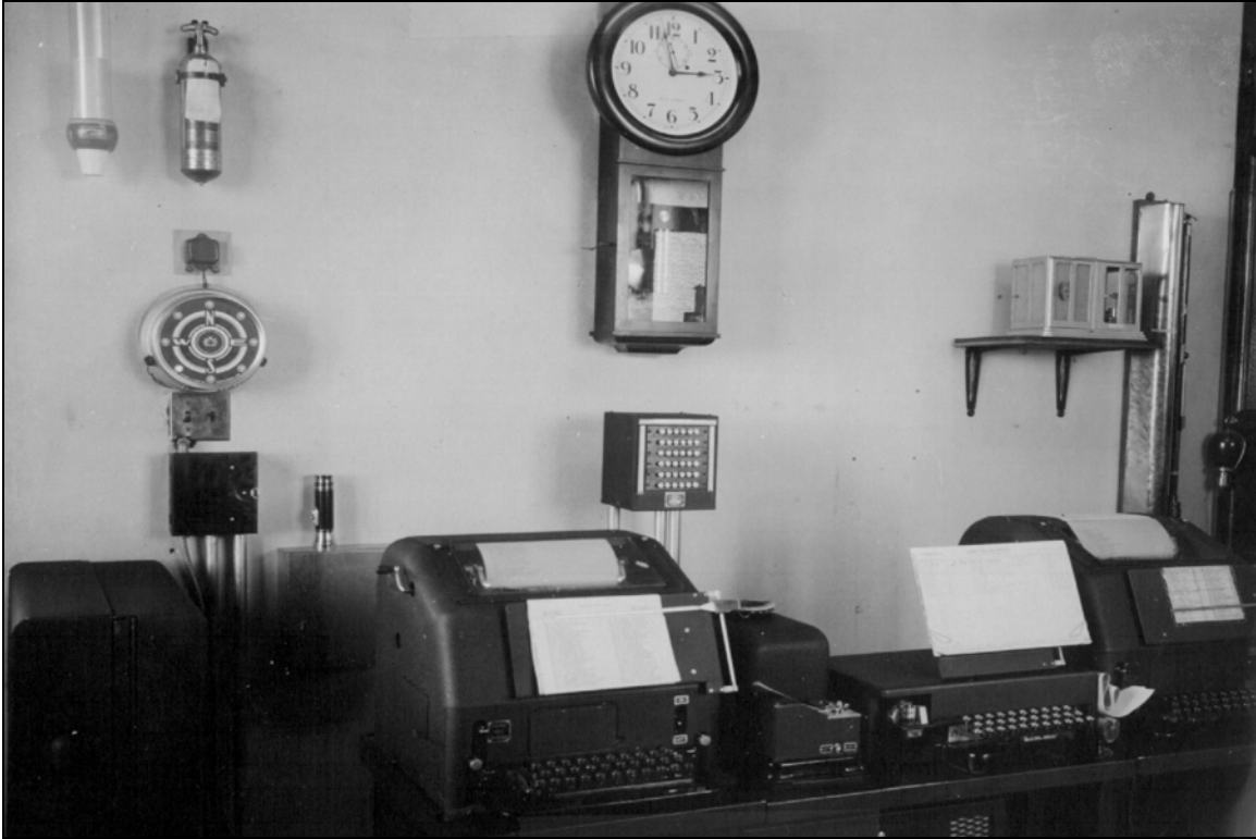
Figure 19. CAA Observatory and communications room in the Administration and Hanger Building (picture taken Oct 1942). Mercurial barometer and barograph on the wall at the far right of the picture. From the official station history files at the National Climate Data Center.
