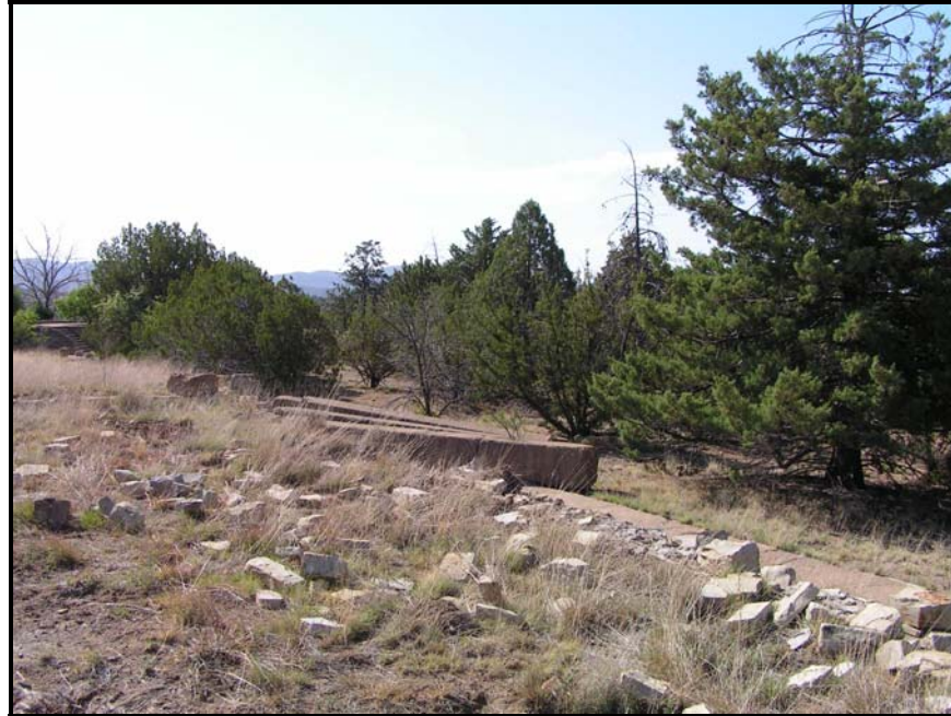
Figure 10. Front foundation of the second Fort Bayard hospital (view is southeast). First hospital was located to the right and down the knoll. Photograph by author (August 2005).
