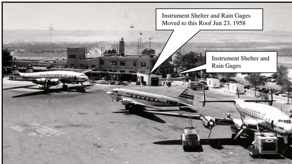
**Figure 30. Location of weather instruments with respect to airplane ground traffic (circa early 1950s). View is northwest. From the Albuquerque Museum.**
