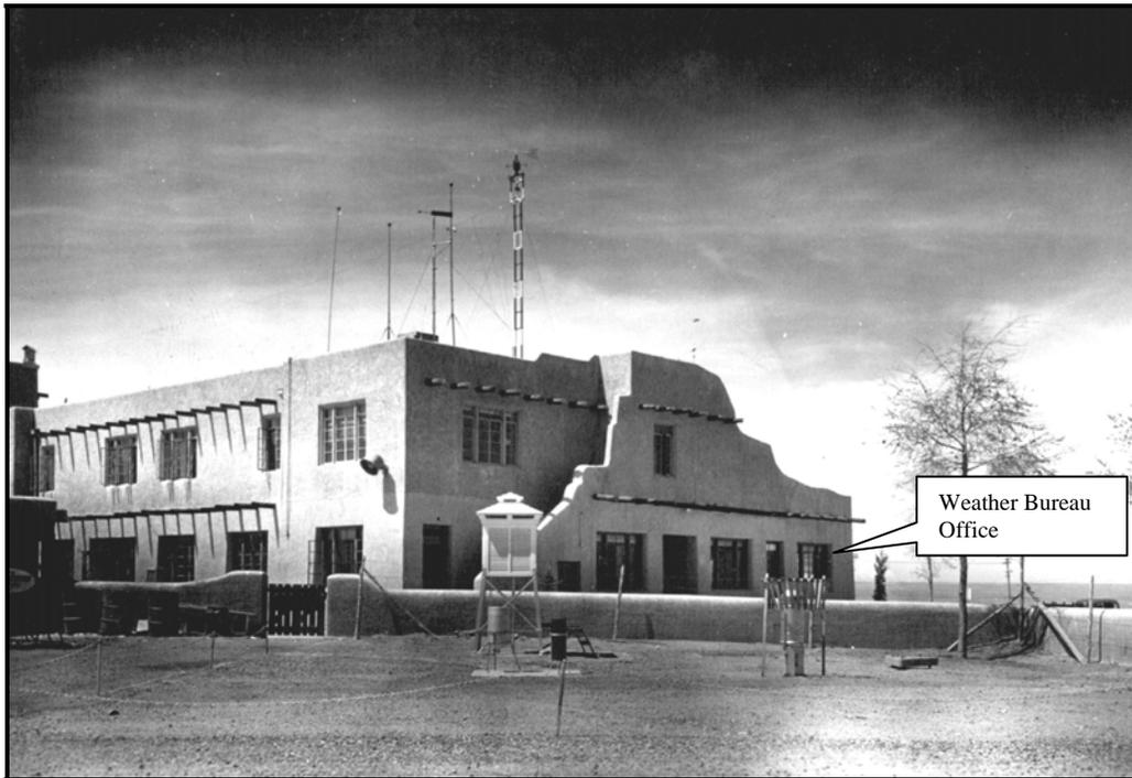
**Figure 24. Instrument shelter, rain gages, and wind instruments at the Municipal Airport Administration Building on 7 April 1944. View is southwest. From the official station history files at the National Climatic Data Center.**
