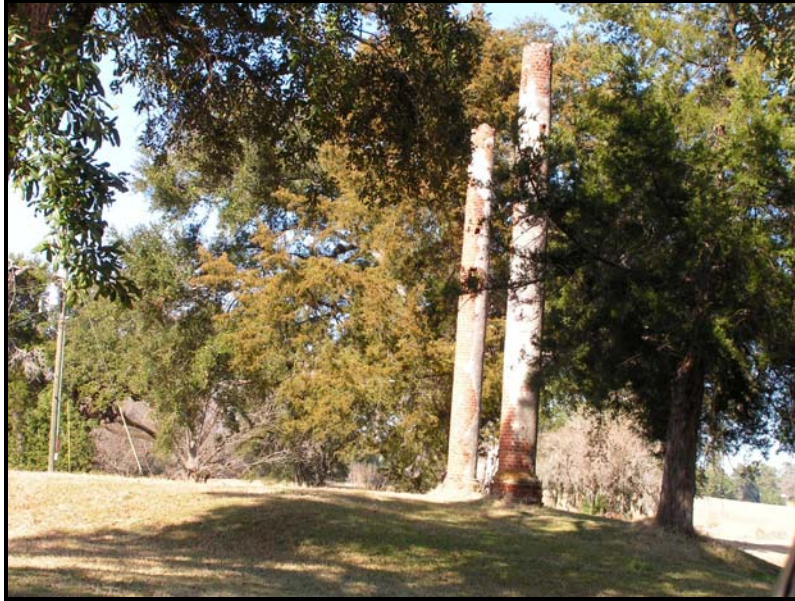
Figure 14. Columns of the Dunbar house. View is toward the west. Photograph made by the author.
