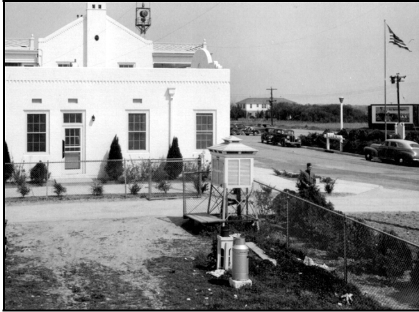
Figure 30. Instrument shelter (new shelter) and rain gages on the west side of the Administration Building at the Jackson Municipal Airport (11 April 1942). Standard rain gage belonged to the Weather Bureau and the weighing rain gage was the property of the U.S. Engineers, Flood Control Section. View is east southeast. From the official station history files at the National Climatic Data Center.
