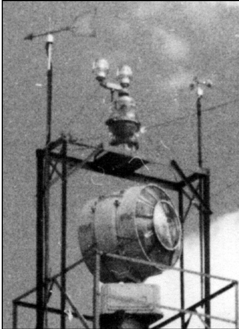
Figure 37. Anemometer and wind vane on top of the beacon tower at the Jackson Municipal Airport (circa 1940). View is northwest. From the official station history files at the National Climatic Data Center.
