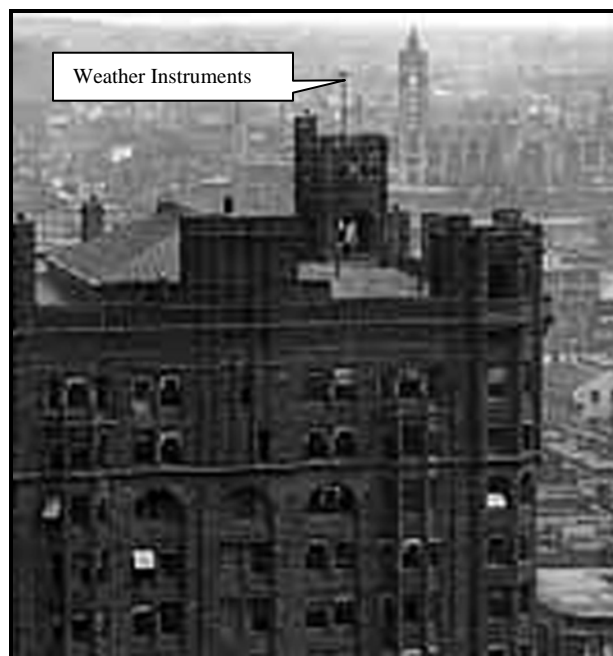
Figure 27. Wind instruments on the Metropolitan Life Building (Guaranty Loan Building) in 1925. View is toward the east. From the Minnesota Historical Society.
