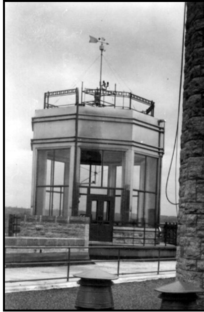
Figure 36. Anemometer and wind vane on top of the Airport Administration Building Control Tower on 1 September 1941. Direction of photograph is southwest. Photograph taken 1 September 1941. From the official station history files at the National Climatic Data Center.
