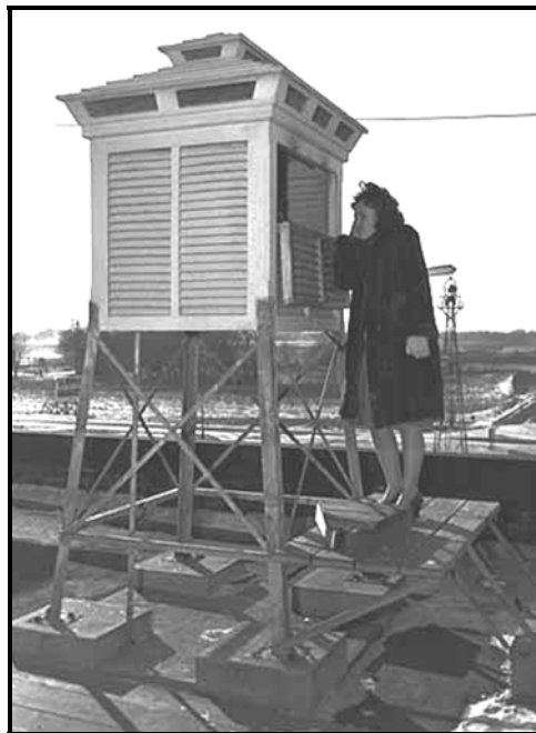
Figure 44. Instrument shelter on the roof of the Wold-Chamberlain Administration Building (circa 1945). View is southwest. From the Minnesota Historical Society.
