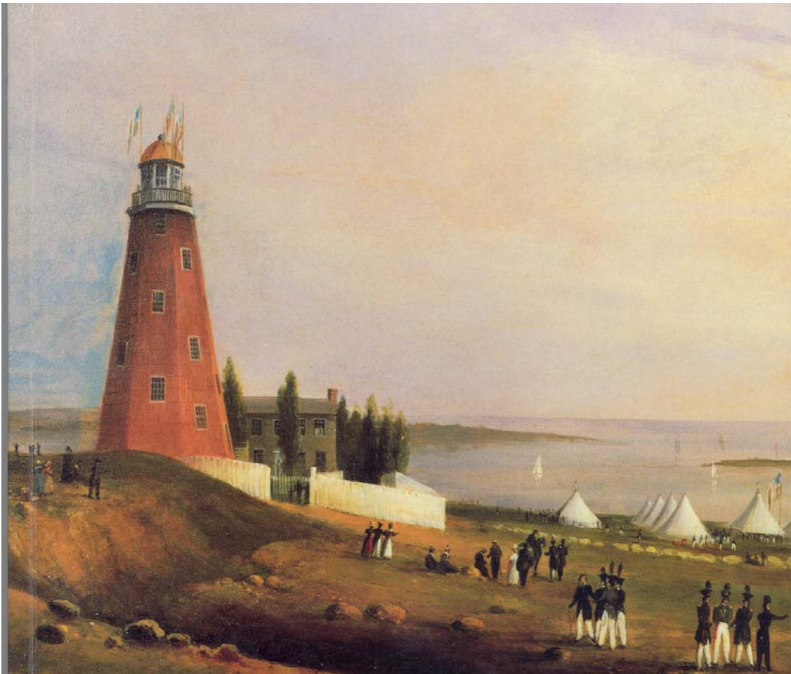
Figure 2. The Portland Observatory, circa 1820, located near the highest point in the city of Portland, Maine, at 138 Congress Street (current address). From the book Captain Moody and His Observatory by John K. Moulton.
