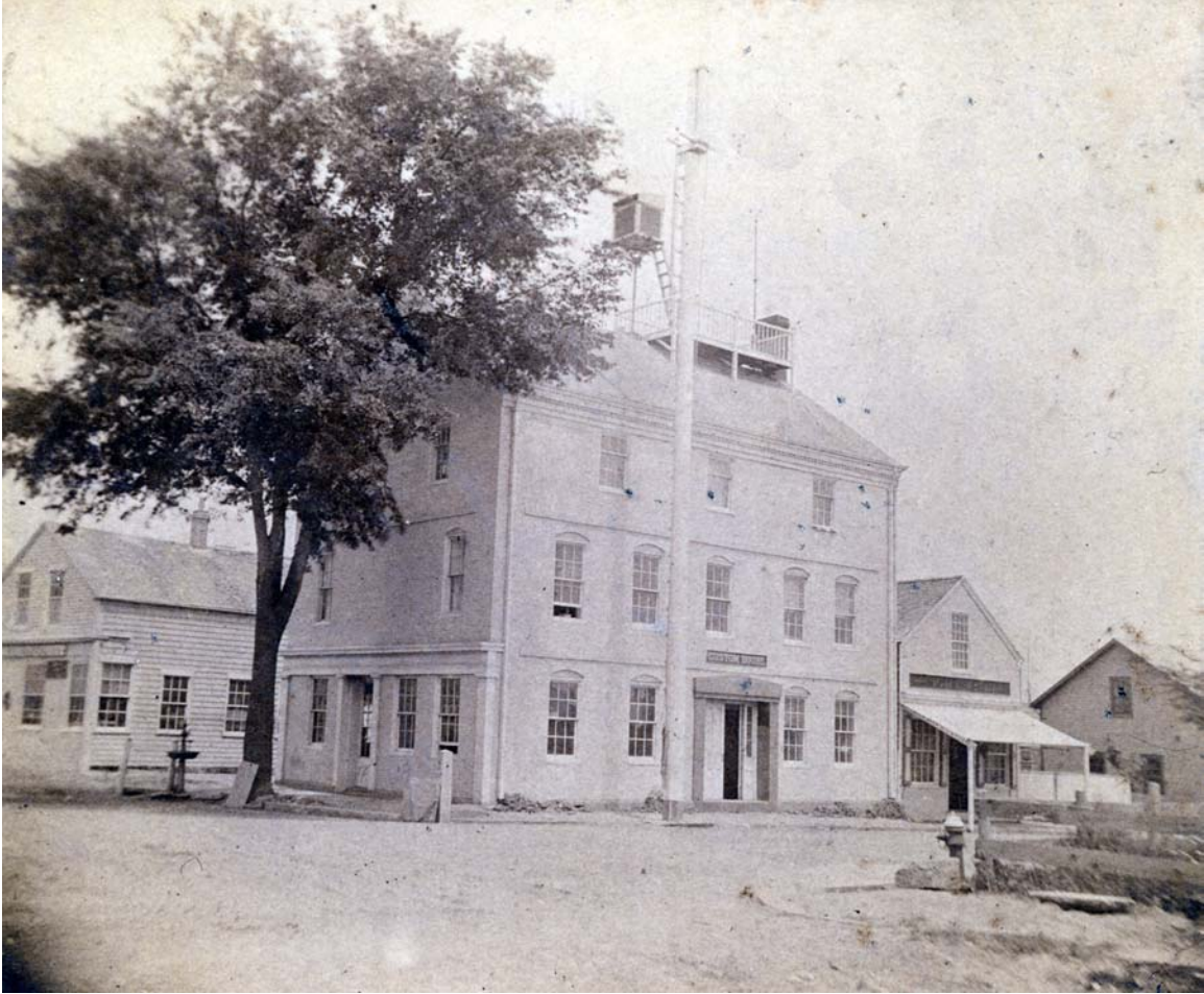
Figure 6. The Pacific Club Building in Nantucket, Massachusetts, circa 1900's. Notice instrument shelter and wind instruments on the roof platform. The Storm Warning Tower appears to have been removed. Photograph from the Nantucket Historic Association (P9558).
