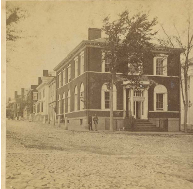
Figure 2. The Pacific National Bank Building in Nantucket, Massachusetts, circa 1860's. Photograph from the Nantucket Historic Association (P6501)
