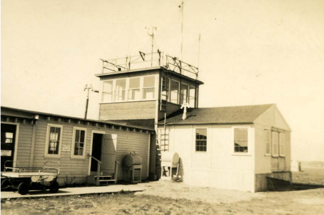
Figure 17. Terminal Building at the Nantucket, Massachusetts, Memorial Airport in 1947. The wind instruments are located on the roof of the building. Photograph from the Nantucket Historic Association (PH2-3-15).
