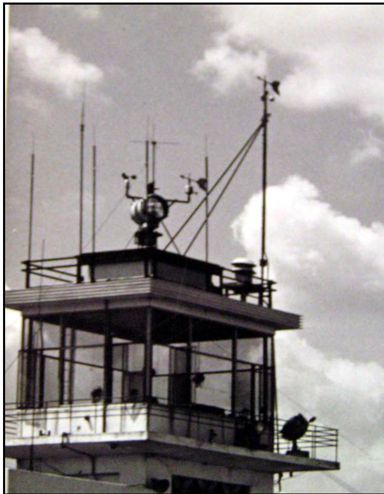
Figure 50. Weather Bureau wind instruments on top of the control tower (mid to late 1940s). View is northwest. From the LSUS Archives—Noel Memorial Library.
