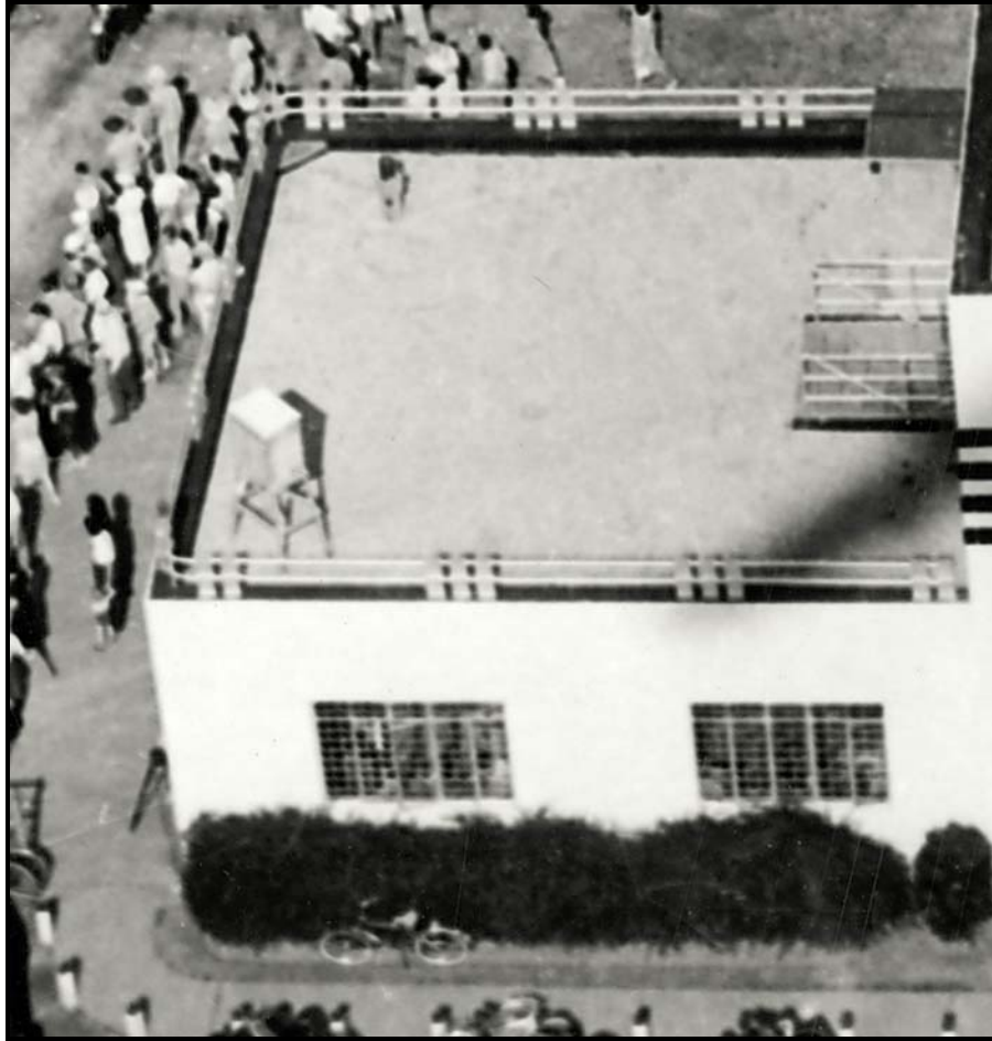
Figure 41. Enlargement of Figure 40 showing instrument shelter and rain gage (1940). North is to the left of the photograph. Note that the door to the shelter faces southeast. From the Shreveport Airport Authority.
