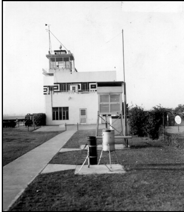
Figure 46. Airport Administration Building, instrument shelter, rain gages, and wind instruments at the Shreveport Municipal Airport (23 April 1943). View is toward the south. From the official station history files at the National Climatic Data Center.
