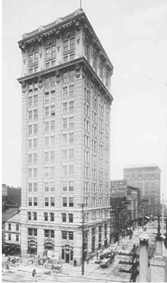
Figure 11. Lincoln Building, 1907, corner of 4 th and Market Streets, Louisville Source: http://www.oldlouisville.com/Ruins/Washington/Washington1907.htm
