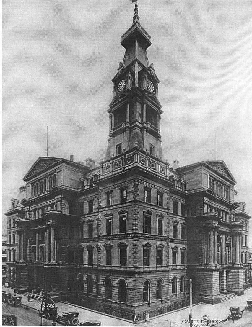
Figure 6. The Post Office and Customs House in Louisville, Kentucky, 1920's Source: http://www.oldlouisville.com/Ruins/PO/PO1920.htm
