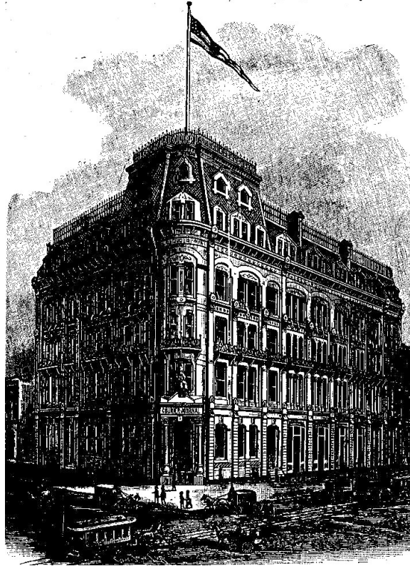
Figure 9. Courier Journal Building in Louisville, Kentucky ca. 1887. Source: Louisville Board of Trade, 1887.
