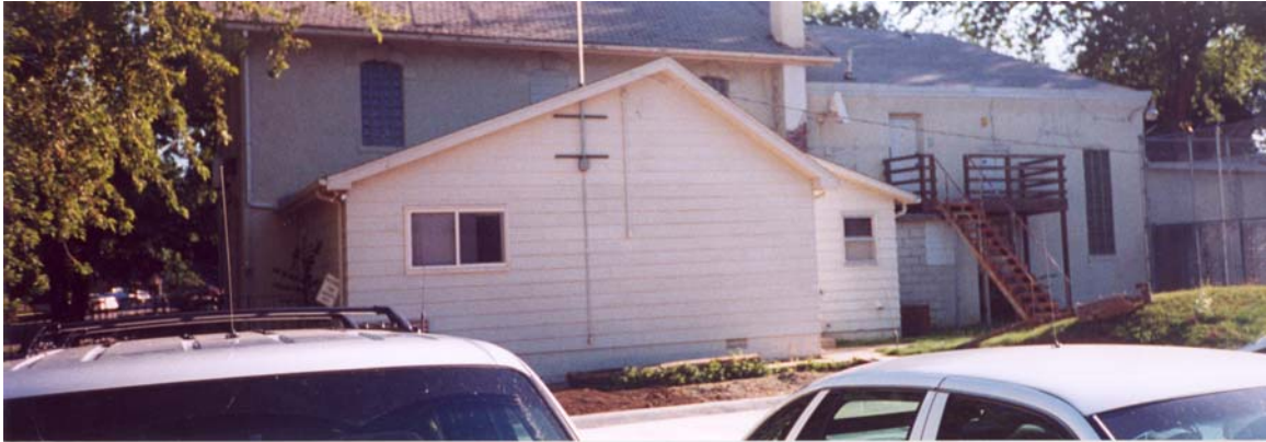
Figure 6. The rear of the “old” county jail on West 6 th Street in Logan, Iowa. The white one-story structure was added in 1987. The weather instruments would have been just off the picture to the right. The building was demolished in 2002 to make room for the new jail. View is looking northeast.
