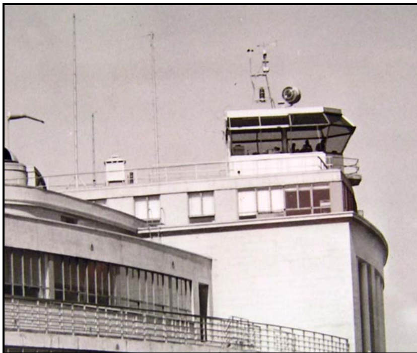
Figure 13. Weather instruments located on the roof of the terminal airport at Washington D.C. National Airport (circa mid 1940s). Instrument shelter is located left of center with an 8 inch rain gage immediately to the right of the shelter. Wind instruments are located on top of the tower. View is towards the north. From the Martin Luther King Jr. Memorial Library.
