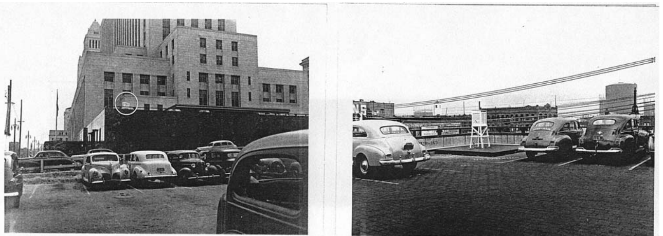
Figure 21. Lower Shelter at Federal Building, 1948
