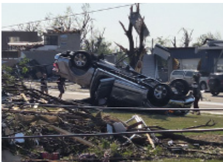
EF-3 tornado damaged structures in Appleton, WI on July 27 (Credit: NWS )
