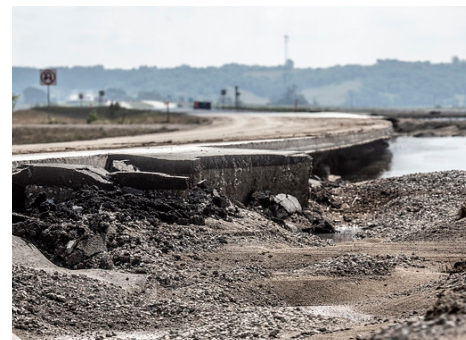
Iowa Highway 2 washed away in early June Missouri River flooding. (Iowa DOT)
