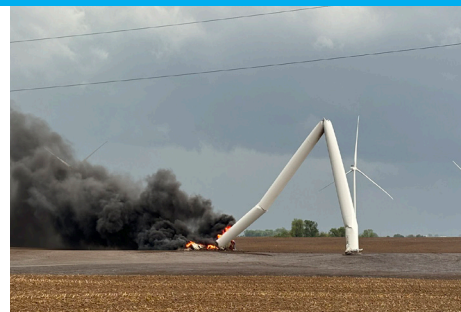
Wind turbine destroyed by the Greenfield tornado in Iowa on May 21 (credit: Colt Forney)
