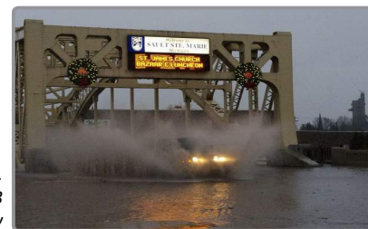
Right: A bridge in Sault Ste. Marie, MI on 11/17/13 Photo courtesy of Jim Lehocky
