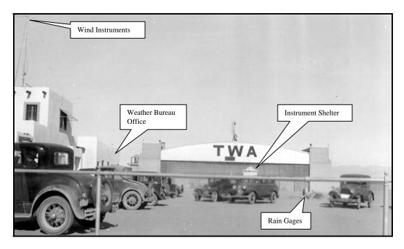
Figure 18. TWA hangar (looking northeast) from the Office and Depot Building (circa 1933). Note location of instrument shelter and rain gages with respect to the parking lot. From the official station history files at the National Climatic Data Center.
