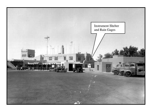
Figure 29. Exposure of instrument shelter and rain gages on 28 August 1956. Note low structures on three sides of shelter and large adjacent hard-surfaced areas. View is northwest. From the official station history files at the National Climatic Data Center.
