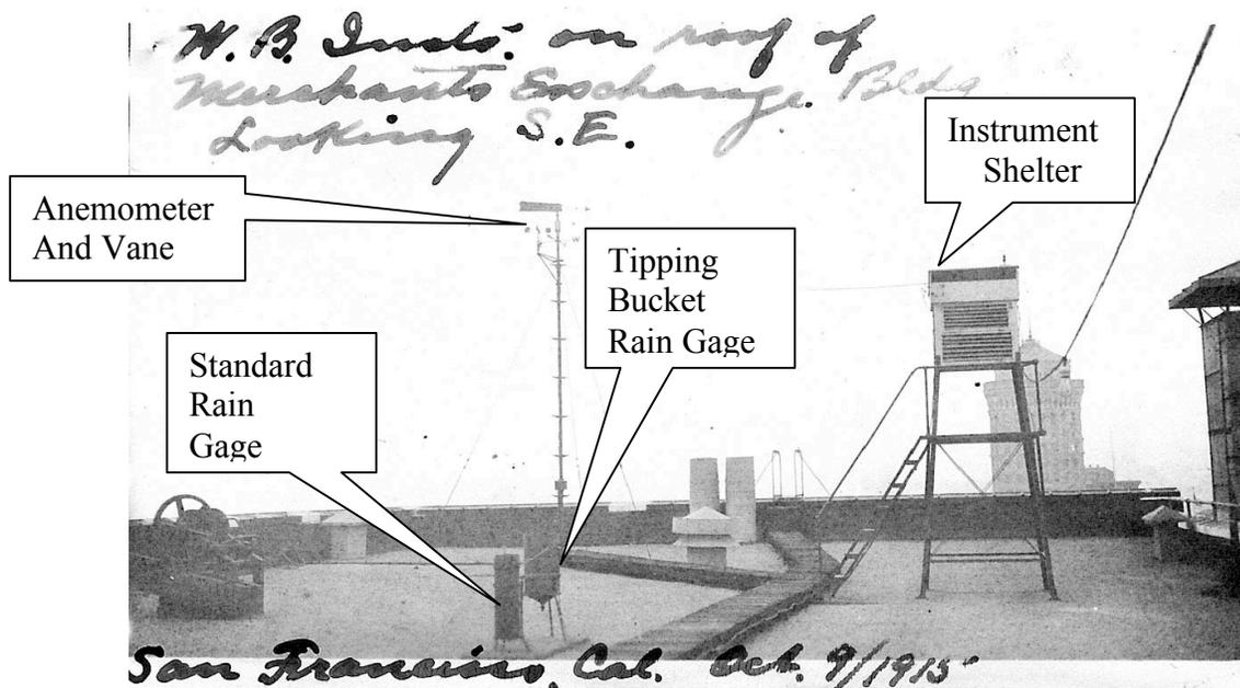
**Figure 9. Rooftop with Instruments, Merchants Exchange Building, 1915**
